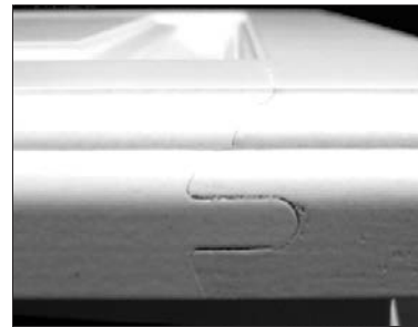
Example of end joint separation
