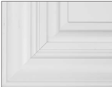
Example of front joint separation
