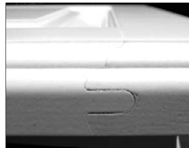
Example of end joint separation
