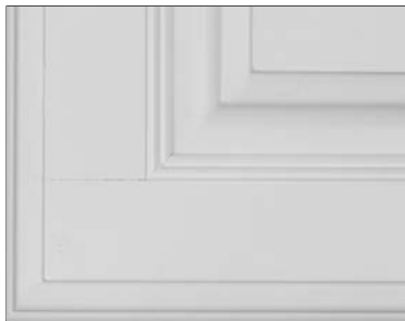
Example of front joint separation
