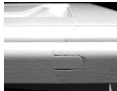
Example of end joint separation
