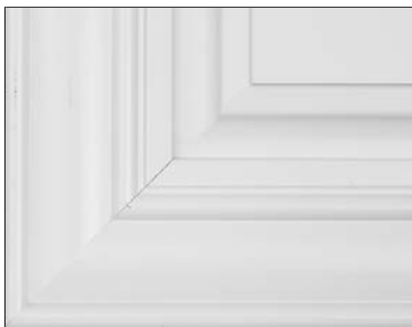
Example of front joint separation
