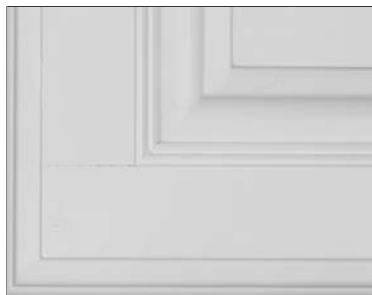
Example of front joint separation
