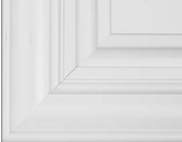
Example of front joint separation
