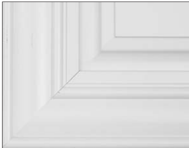
Example of front joint separation
