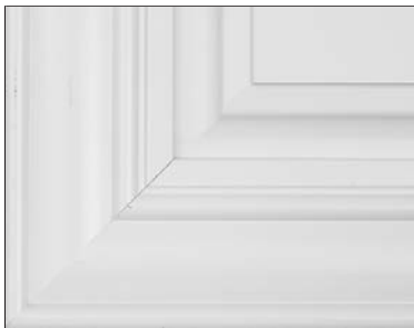
Example of front joint separation
